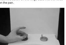
Aim at the holes and adjust the hinge base to make the seat cover and pan match.
